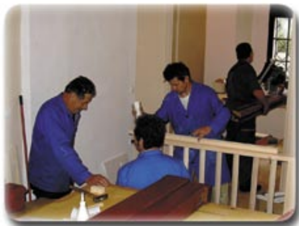
Mizarska in tesarska dela
